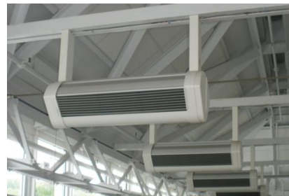
LTG coolwave system with two chilled water coils (Image source – CBPD)
