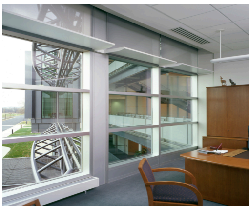
Wausau internal lighting shelf at Armstrong World Industries office in Lancaster, PA. (Wausau, 2017)
