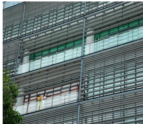
Horizontal louvers on south face of Stecalite, Noida.
