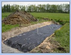
4. Woodchip addition - Digger fills in 5. Bioreactor cover- Depending on 6. Monitoring & maintenance - Check soil type and other local conditions, inflow structures and piping in winter/ a geotextile cover should be installed, spring with higher flow. Maintenance will especially if farming will continue over be site-specific and vary from year to year. bioreactor. Top the bioreactor with soil.
