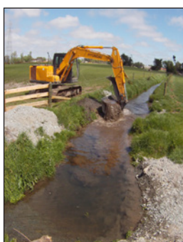
Digging sediment traps with the Waimakariri District Council drainage engineering team in 2014.
