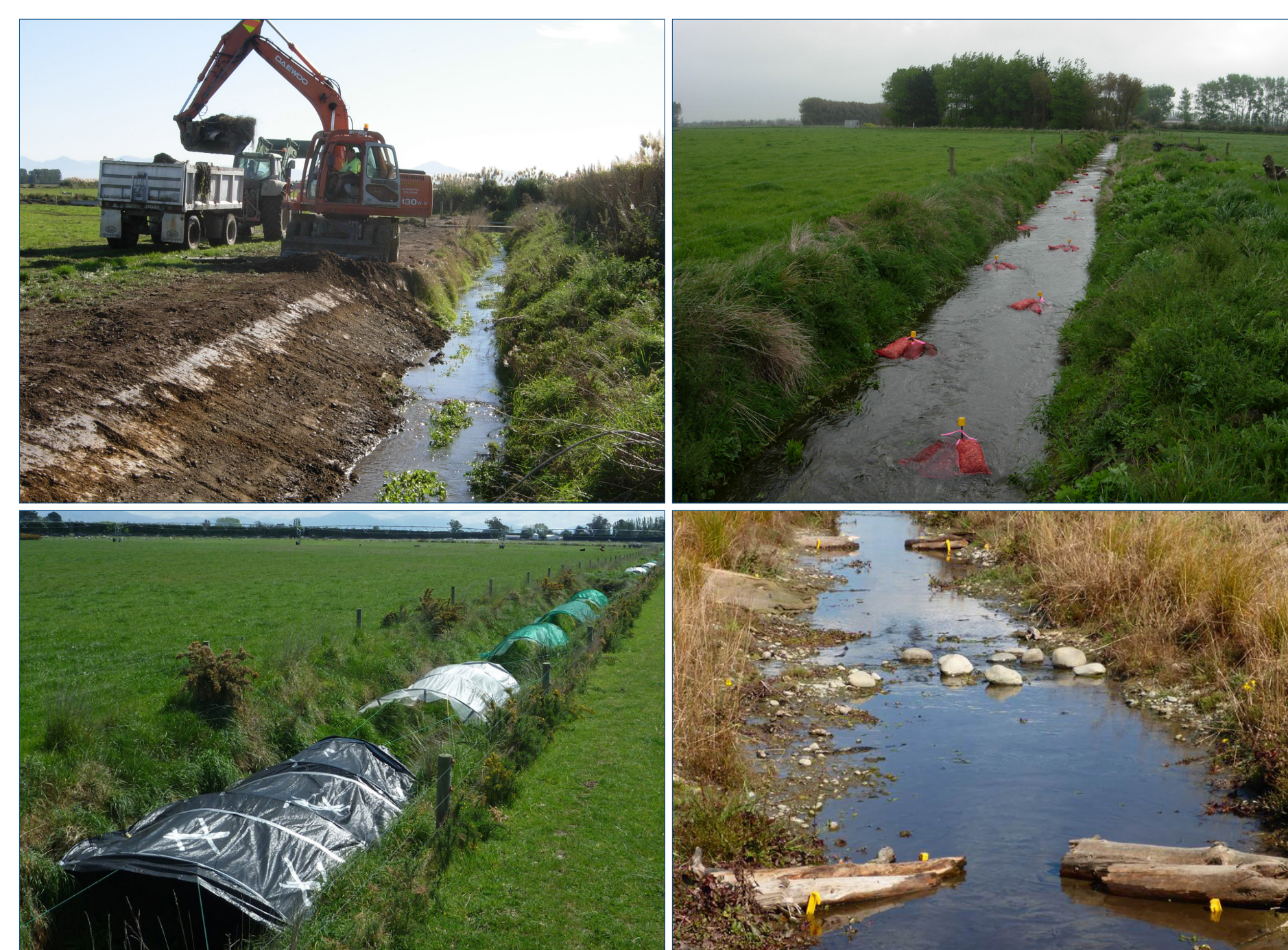
Trialling the restoration tools: rebattering the banks, organic matter additions, shading macrophytes, and creating in-stream habitat.
