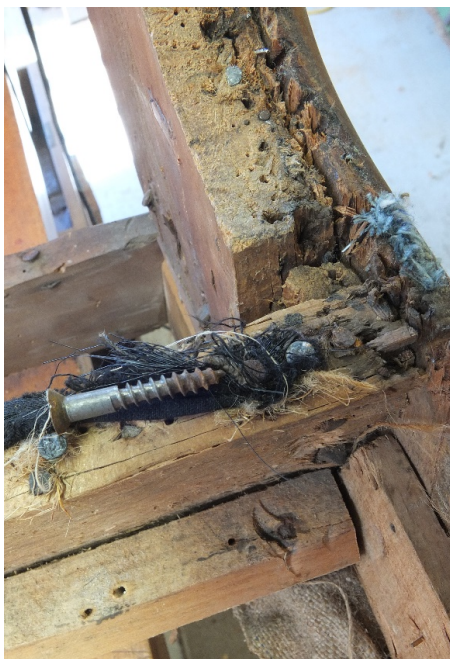
FIG 8 (left): Original screw with tapered gimlet-point.
