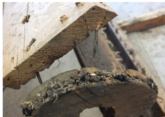
FIG 8 (left): Original screw with tapered gimlet-point.
