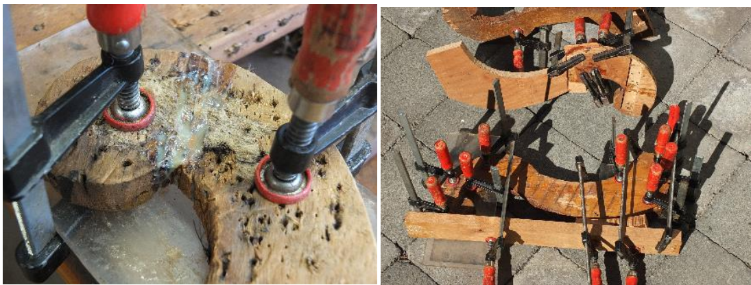
FIG. 5 (left): Epoxy resin was used to support fractured kauri framing substrates.
