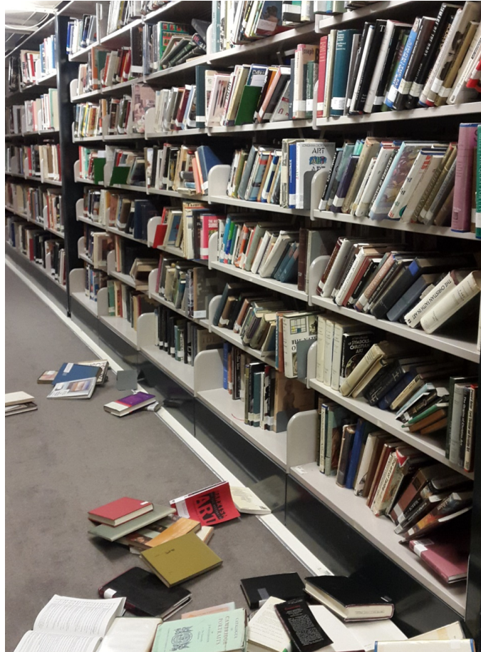
FIG. 18: These shelves are part of a static range at the end of ranges of mobile shelves. The arrow indicates the transition between the bays with anti-slip shelf liners and the five bays (in the foreground) that have no shelf liners. The books on the background shelves stayed upright and none fell from the shelving (courtesy Alexander Turnbull Library).
