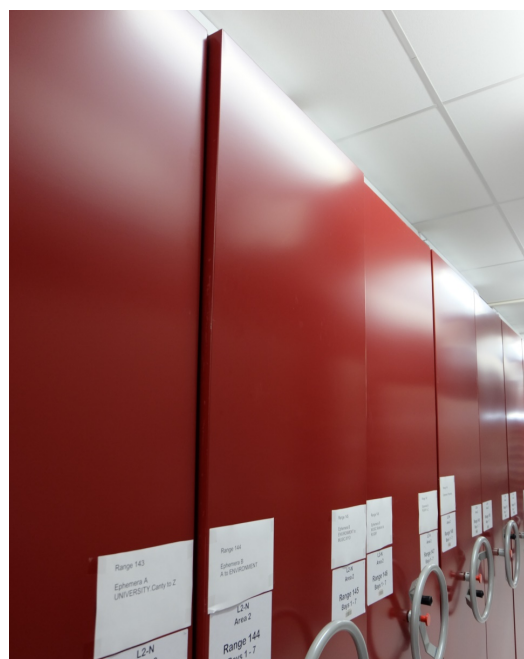
FIG. 7: The partially failed range in a level 2 store was out of alignment with adjacent ranges. The engineers recommended the installation of cross bracing to improve seismic resilience (courtesy Laura Mirebeau).
