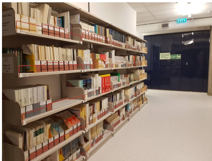
FIG. 9: Safety bars were installed on shelving along all collection store egress routes to protect staff from falling items and to ensure egress routes remained viable in a major earthquake (courtesy Alexander Turnbull Library).
