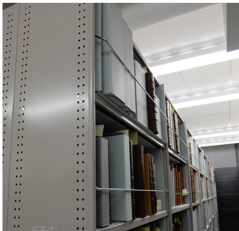
FIG 17: Seismic restraints on shelving prevented the books that had shimmied forward on the shelf from falling onto the floor (courtesy Alexander Turnbull Library).
