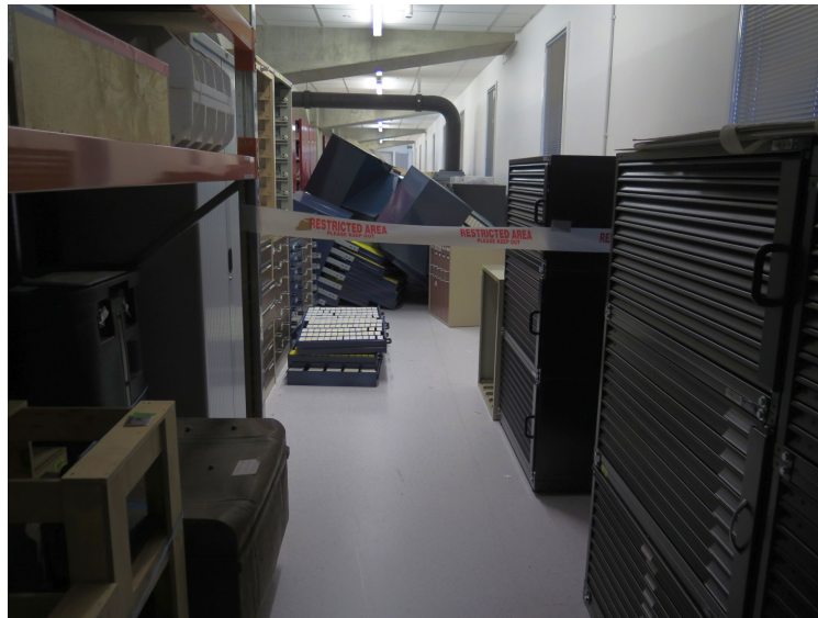
FIG. 6: Fallen two-part microfilm cabinets blocking the aisle and cordoned off (courtesy Margaret Morris).
