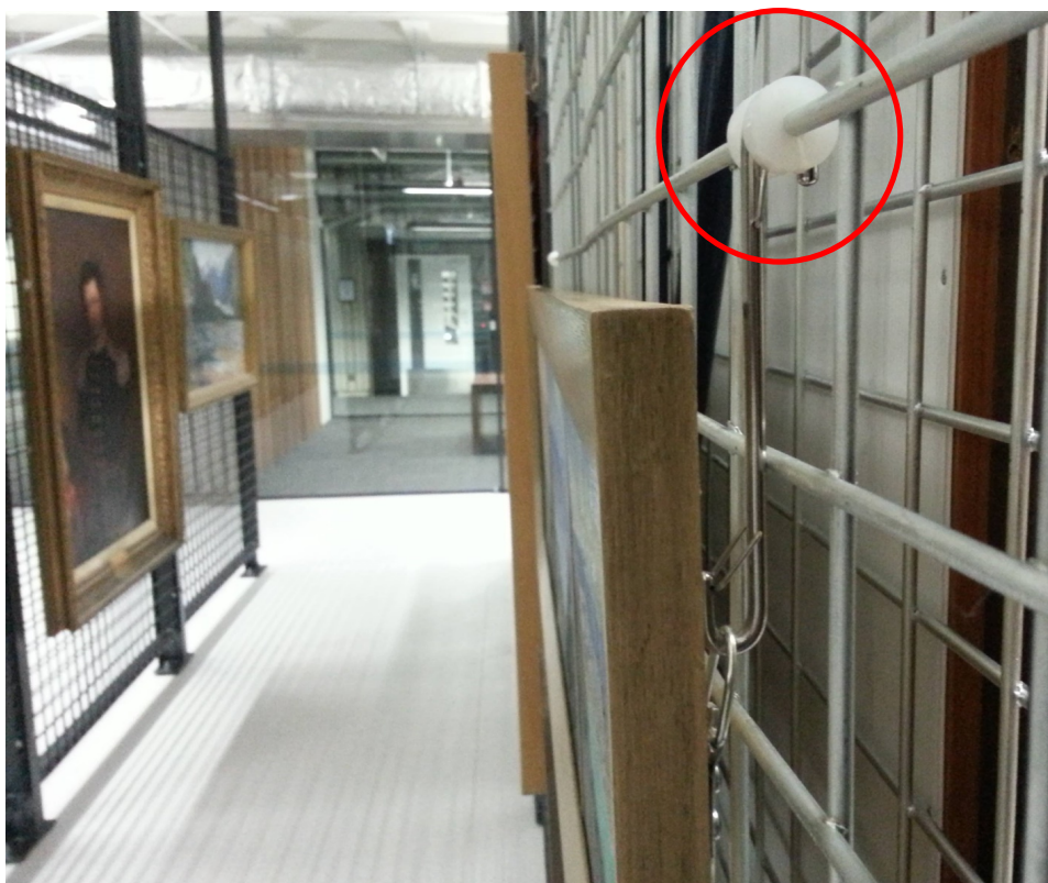
FIG. 3: The silicon bumper (circled) on each hanging hook significantly limits movement of the hook which protects the framed items from excessive movement during seismic activity (courtesy Margaret Morris).
