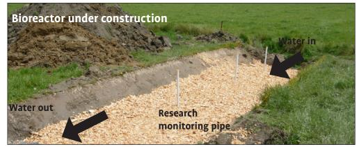
**Why woodchips?** A practical, affordable, sustainable & long-lasting (10-15 years) carbon source. Untreated woodchips either hardwood or softwood, ~ 2.0cm in size (to avoid compaction when in bioreactor), are best.
