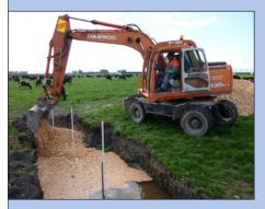
bioreactor with wood chips.
