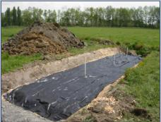
bioreactor. Top the bioreactor with soil.
