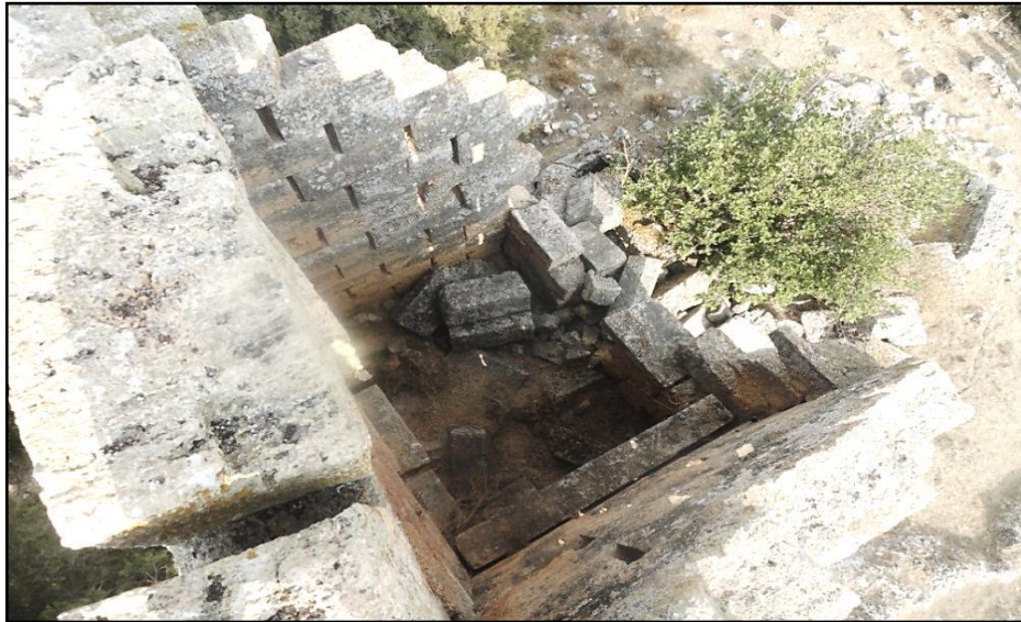
Figure 4.31: Qasr Aqeela: The string course that separated the two levels.
