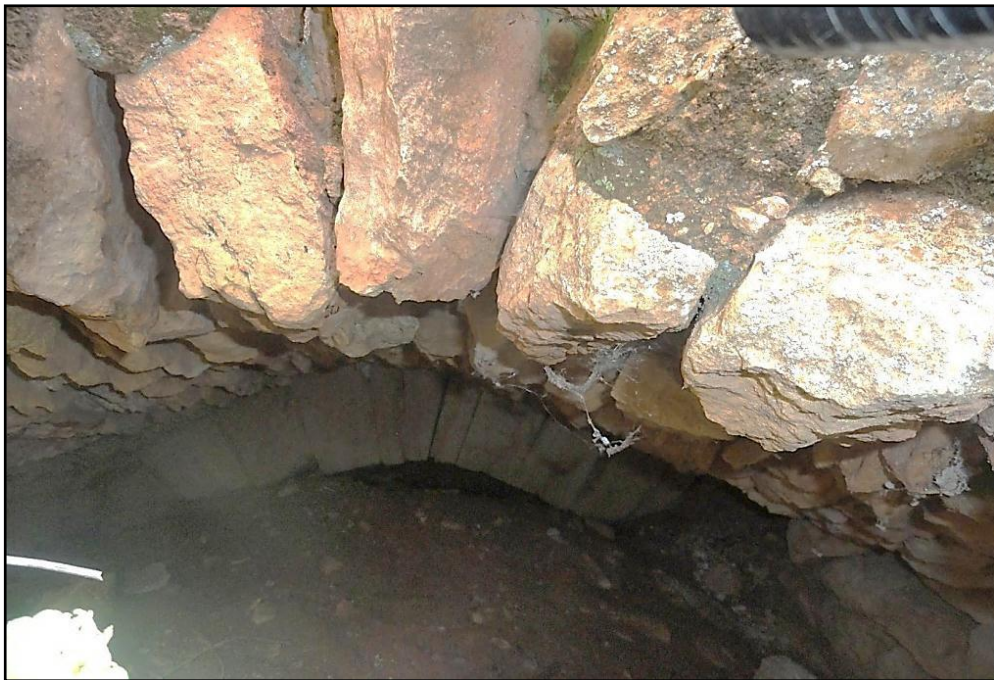
Figure 4.27: Qasr al-Akrout al-Warrany 2: The vaulted chamber of the Ground floor.
