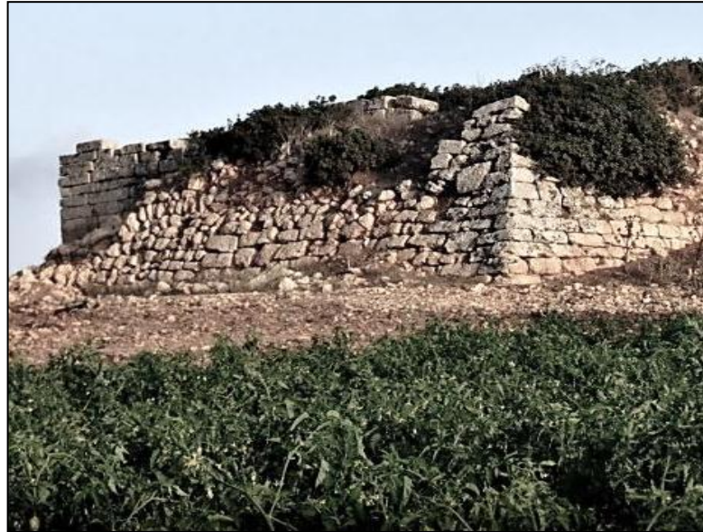
Figure 4.8: Qasr Az-Zaaroura: An example of the sloping revetments.
