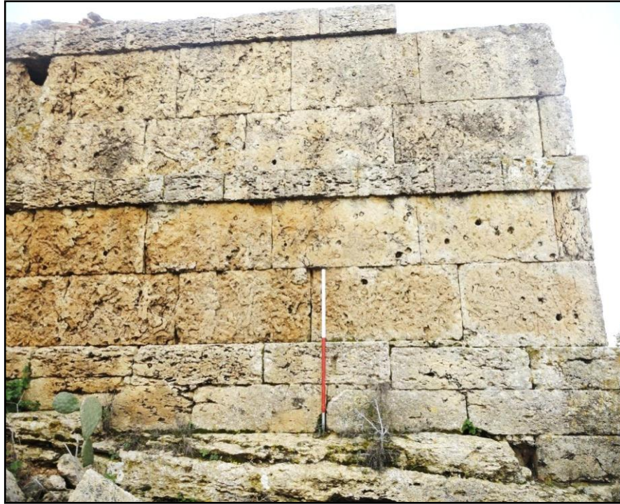
Figure 9.78: Siret et-Tauma 4: North wall shows type of masonry and string courses, looking south. Scale 1.
