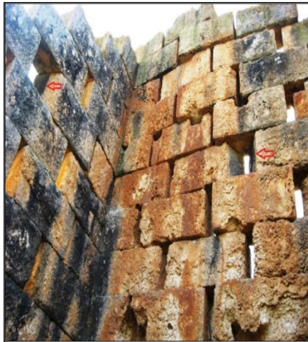
Figure 5.6: Qasr Aqeela: The window slots. Figure 5.7: Qasr Aqeela: Gaps between the blocks.
