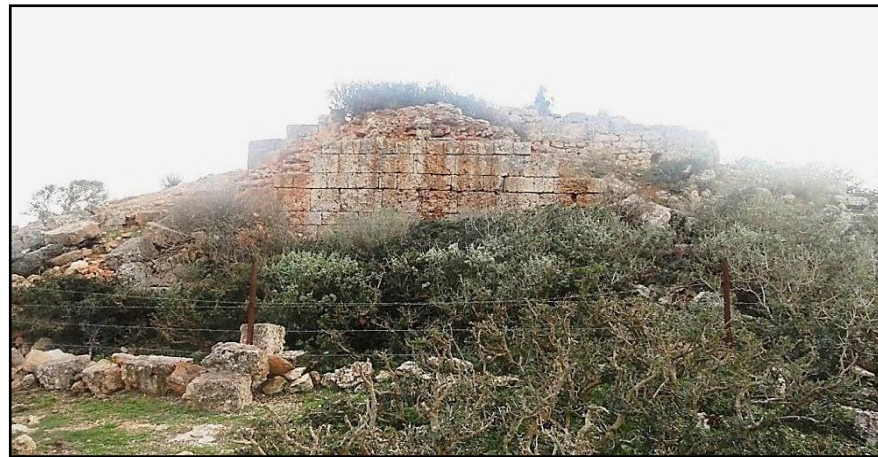
Figure 4.13: Qasr Sidi Bu-Argoub: Ashlar masonry utilised in the revetment.
