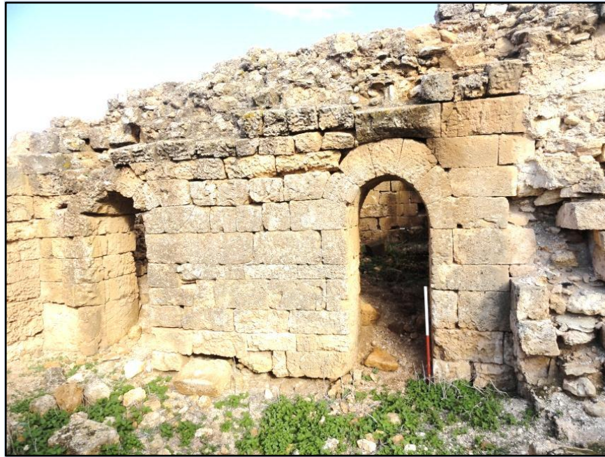
Figure 4.7: al-Qasr al-Hamar: The use of rubble masonry in the upper storey. Scale 1m.
