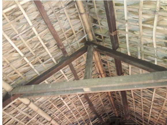
Figure:21 Main truss support (Source: author)
