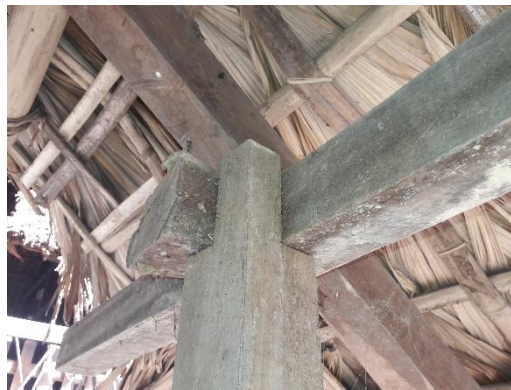
Fig-17: Joinery between beam and column (Source: author)
