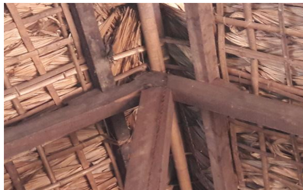
Figure:21 Main truss support (Source: author)
