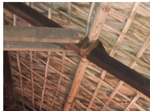
Fig-23: Purlin-rafter binding (Source: author)
