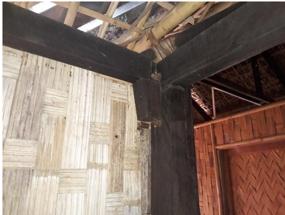
Fig-22: Wall-frame connection (Source: author)
