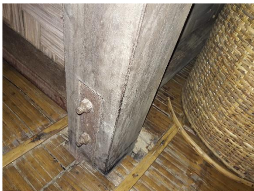
Fig-20: Floor-column connection (Source: author)
