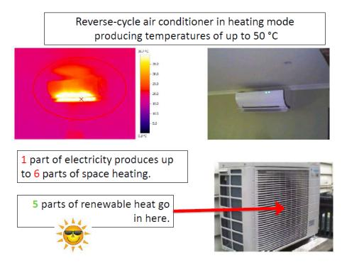
Figure 17: - A reverse-cycle air conditioner in heating mode harvests renewable-ambient heat [source: Tim Forcey<sup>109</sup>].
